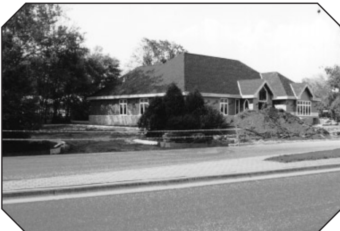
Parking lot on the west side of building, prepared for laying of blacktop
